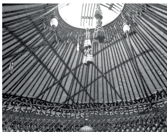
Figure 3 Structure of Kazakh felt tent
